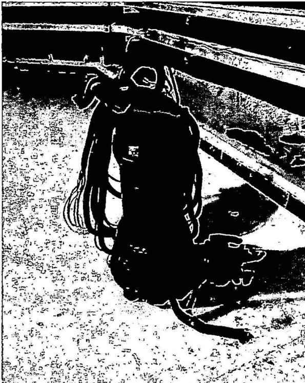
Bomba sumergible tipo: ABS XFP100G-CB1.6
